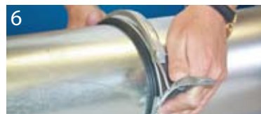
6 Snap QF clamp over O-ring and one end of slip duct.
