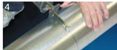
4 Cut the duct.
