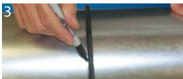
3 Use O-ring provided and mark for cut.
