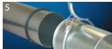
5 Put O-ring on cut duct, slide slip duct over cut piece of duct.
