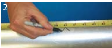
2 Mark distance to be spanned less 100 mm.
